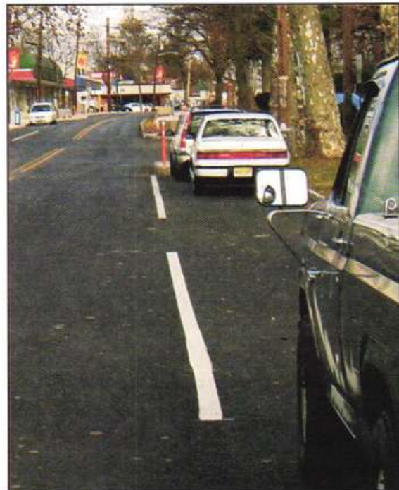
Figure 3.2.2.10: Edge line before curb extension.
