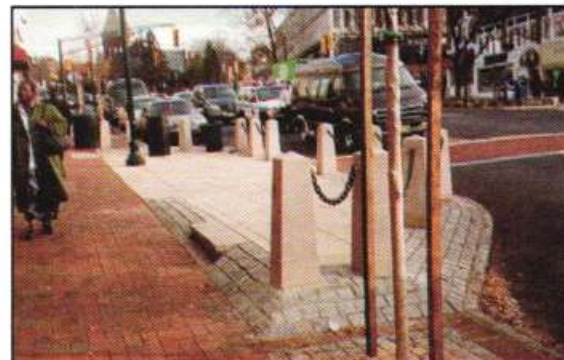
Figure 3.2.3.18 Curb extension with bollards.
