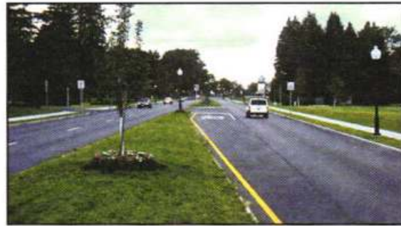
Figure 3.3.4.7: Twenty-three foot raised median with turn bays.
