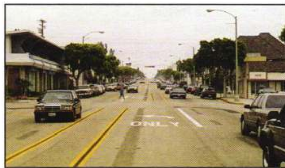
Figure 2.6: Nonconforming median, Los Angeles, California.
