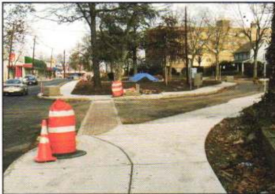
Figure 3.2.2.14: Entrance to Old South Avenue.
