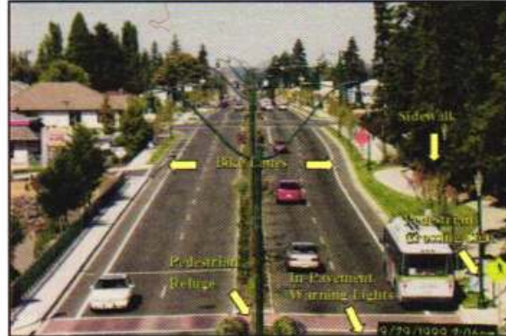
Figure 2.23: Midblock crossing designed for high visibility, University Place, Washington.
