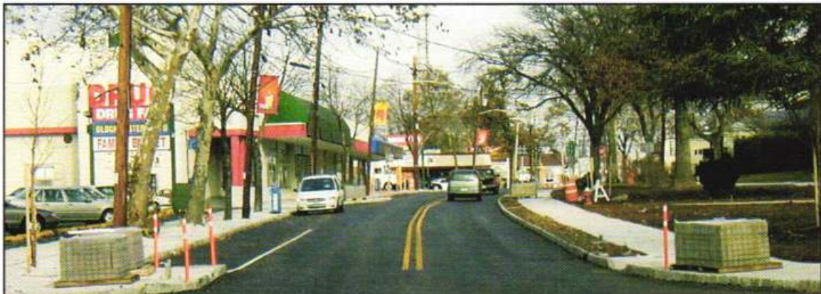
Figure 3.2.2.1: South Avenue construction.
