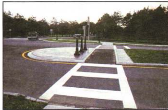
Figure 3.3.4.19: Well-marked crosswalk and accessible median.
