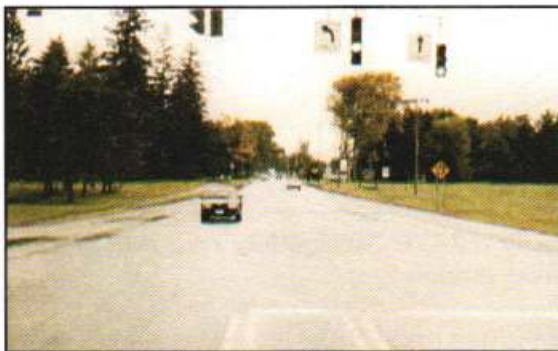
Figure 3.3.4.13: Avenue of the Pines intersection before.
