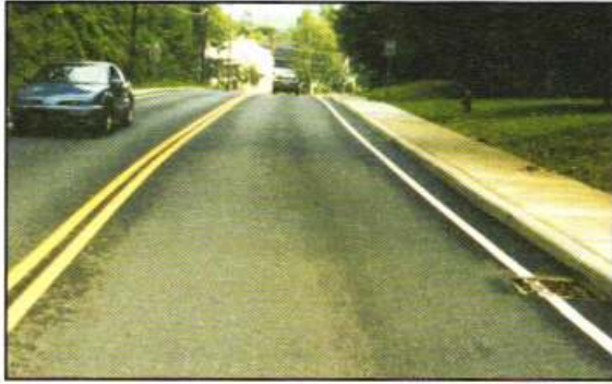
Figure 3.3.1.5: Drainage grate and edge line.
