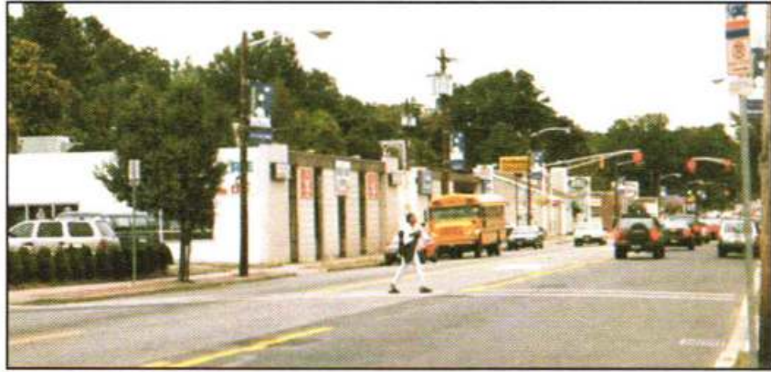
Figure 3.2.1.13: Existing uncontrolled crosswalk.
