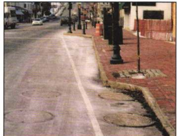
Figure 3.2.3.11 Edge lines where street width is reduced in segments.
