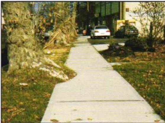
Figure 3.2.2.18: Sidewalk at tree.
