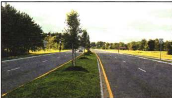
Figure 3.3.4.5: Twelve-foot raised median.
