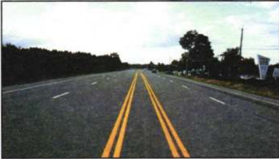
Figure 3.3.4.3: Four-foot flush median.
