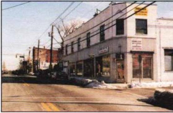
Figure 3.2.1.8: Existing at Ohio Street.
