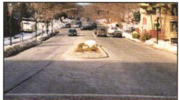
Figure 3.2.3.12 Raised median as a gateway into town.
