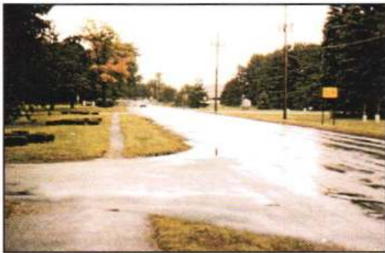
Figure 3.3.4.17: Former sidewalk condition.
