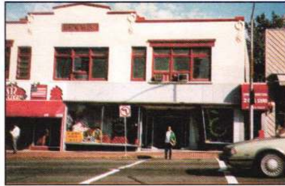
Figure 3.2.3.15 Before crosswalk at Academy Street.
