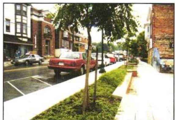
Figure 3.3.5.15: MD 144 through Hancock after.
