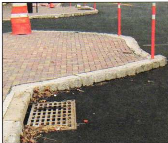
Figure 3.2.2.8: Inlet at curb extension.
