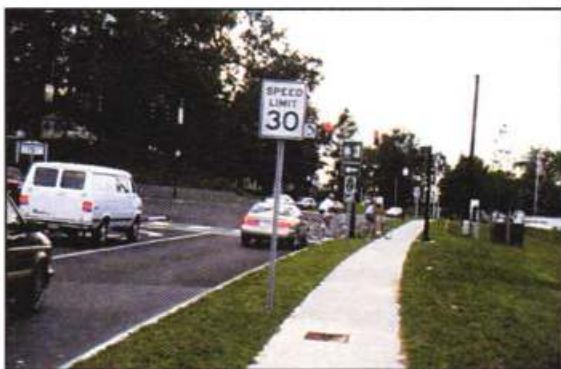
Figure 3.3.4.18: New sidewalk condition.
