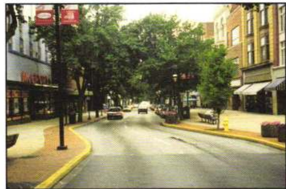
Figure 2.35: Traffic calmed main street in York, Pennsylvania.
