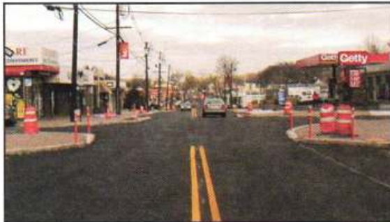
Figure 3.2.2.7: Typical curb extensions.
