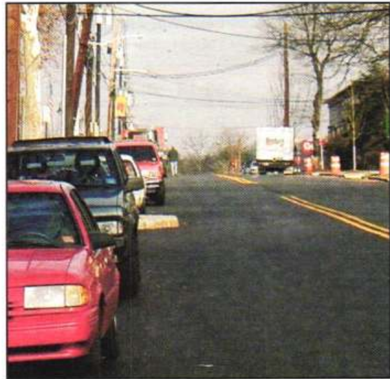
Figure 3.2.2.9: Curb extension poking out between parked cars.
