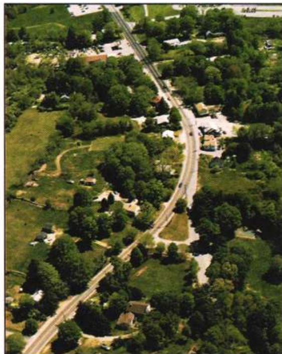
Figure 3.3.2.10: Curve at Tatnic Road.
