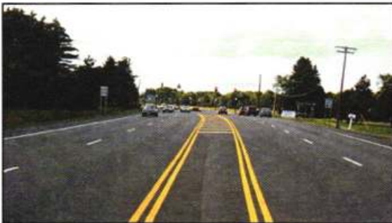
Figure 3.3.4.4: Twelve-foot flush median.
