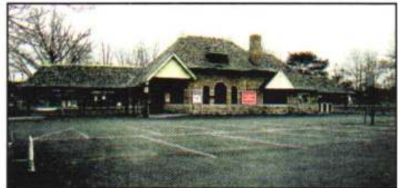
Figure 3.2.2.21: Former train station.
